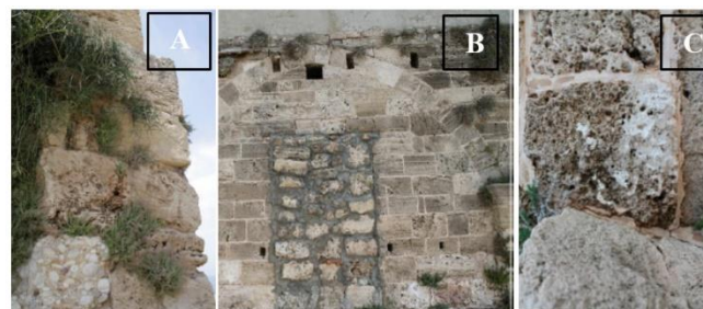
Figure 2: Images taken at site in Tyre City showing Structural and Physical Changes (Problems). (A): Spread of Plants; (B): Appearance of Cements sheets on main elevations; (C): Masonry and Stone Problems (appearance of Black colors, Bacteria, holes...) (Source: Author)
