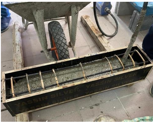
Figure 1. Vibration of concrete inside the molds.
