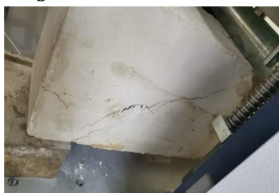
Figure 11. Beam B3 (I-section) Cracks
