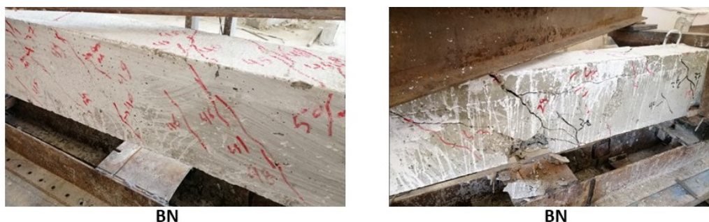
Figure 7. The Cracks Propagation in BN Beams
