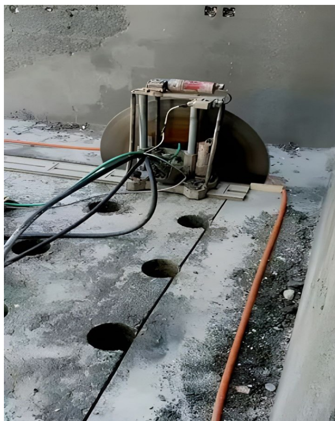
Figure 7. Creation of Slab Openings to Facilitate Concrete Casting During the Rehabilitation of the Damaged Load-Bearing Wall
