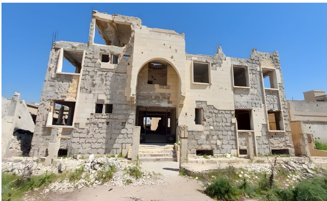
Figure 2. The Front Elevation of the Building.
