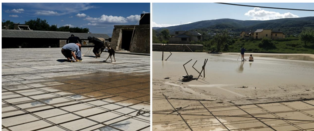
Figure 5. Upper Slab Strengthening Procedure Adopted for Reinforcing the Damaged Floor System
