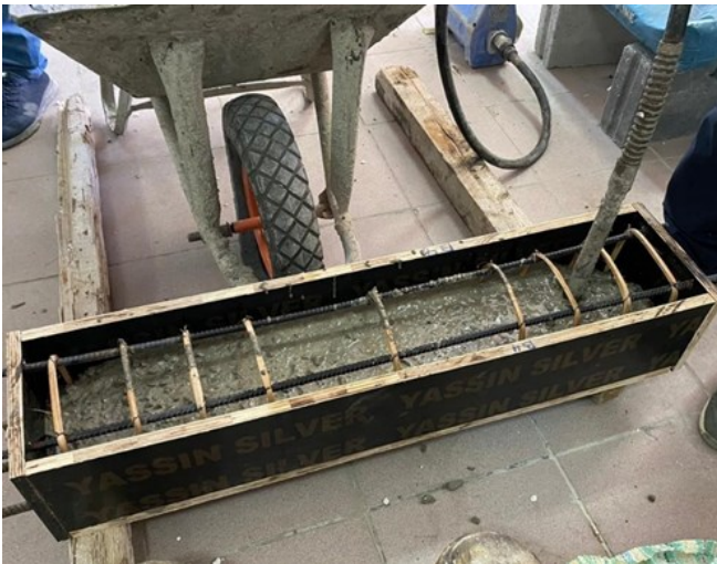
Figure 1. Vibration of Concrete Inside the Mold
